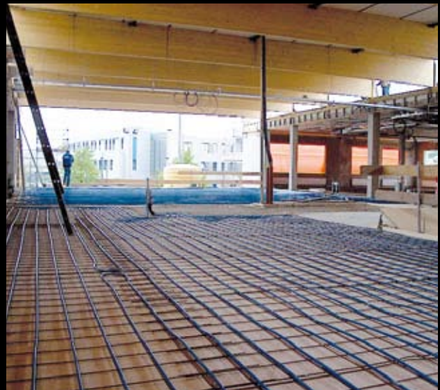
Montage op netten school te Ede
